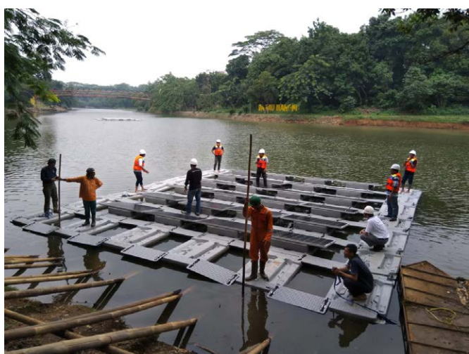
Proses Instalasi PLTS Bi-facial Bi-facial Solar Power Plant Installation Process
