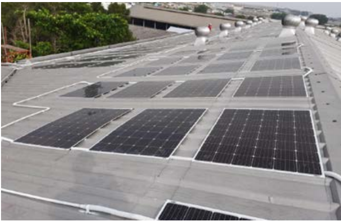
Instalasi J-Leaf di Atap Gedung Industri Kawasan Bekasi J-Leaf Installation on Bekasi Industrial Building Rooftop
