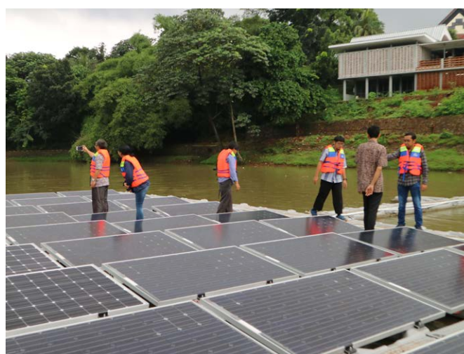
Proses Instalasi PLTS Bi-facial Bi-facial Solar Power Plant Installation Process
